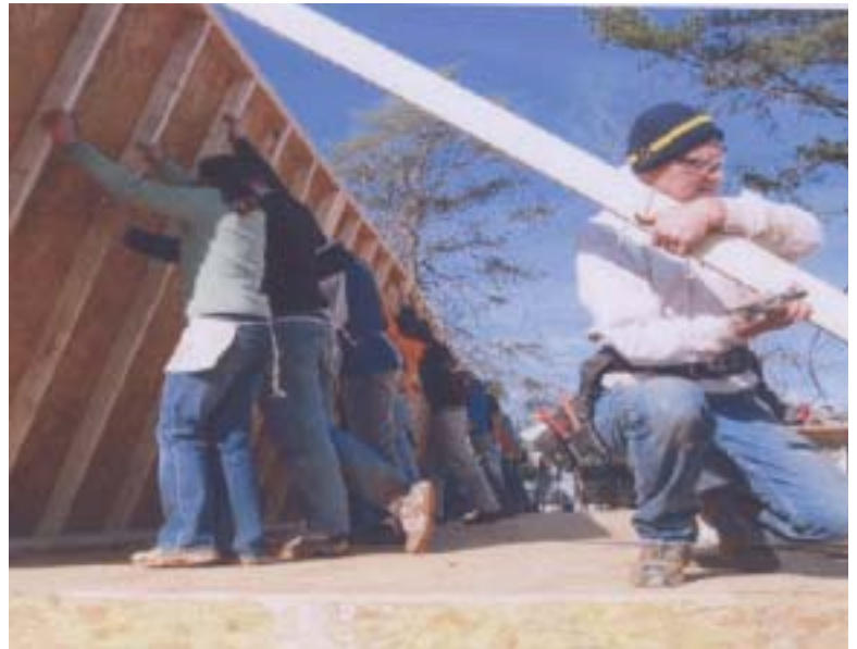
Below: Up go the walls on Deb's Habitat house.
